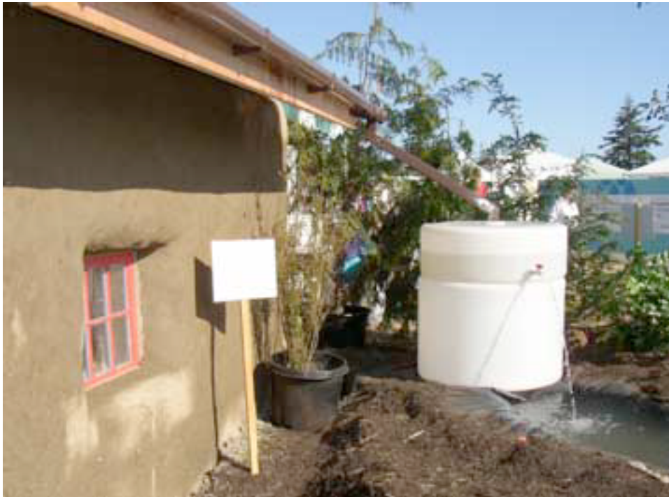
Cob and straw bale building with rainwater catchment system.
